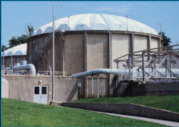
Williamsburg WWTTP Hampton Roads Sanitation District Williamsburg, Virginia, EUA
